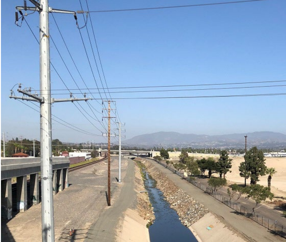
Anaheim Lake site from Orangethorpe overpass, showing Atwood Channel and existing 66 kV SCE overhead line (May 4, 2022 photo)
