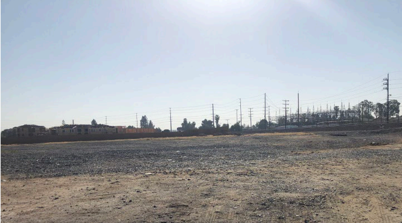
RPU Freeman substation and potential Gibson Street laydown area (May 1, 2022 photo)
