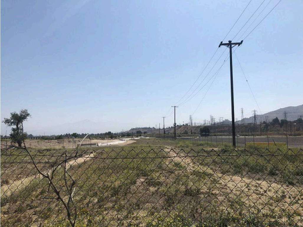
Looking east from potential Santa Ana River substation site towards Vista Substation (May 1, 2022 photo)
