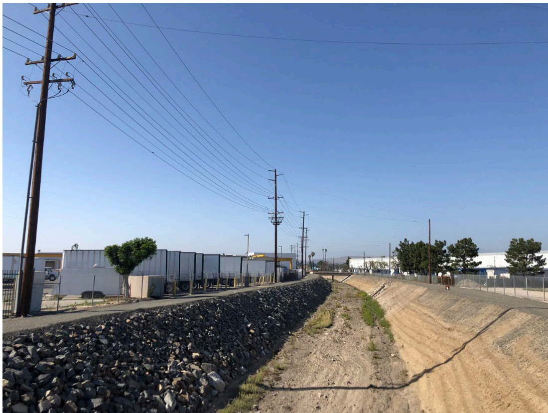
Looking north along Carbon Canyon Diversion Channel and 69 kV APU overhead line (May 4, 2022 photo)
