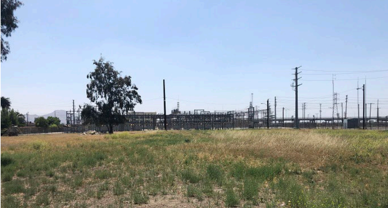
SCE Calelectric substation and potential laydown area (May 1, 2022 photo)
