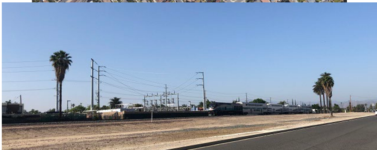
RPU Casa Blanca substation and potential laydown area (May 1, 2022 photo)
