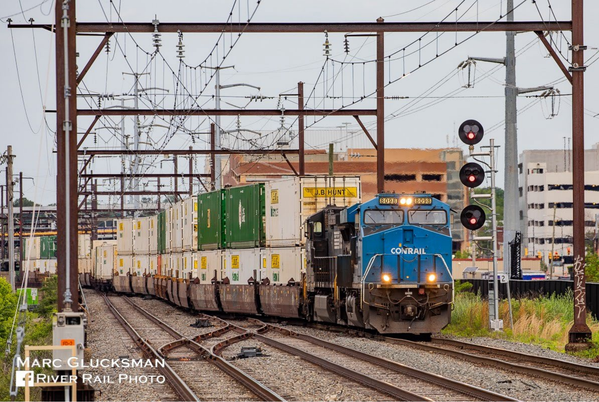
Double-stack container train under overhead contact system (OCS) in Philadelphia area (Class 1 railroads operate diesel powered freight trains under wires on this corridor) 24
