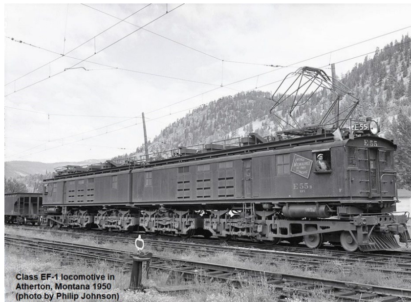
The Milwaukee Road was running electric long-distance freight and passenger trains on 663 miles of electrified track through the Cascades and Rocky Mountains, from 1914 to 1974.
