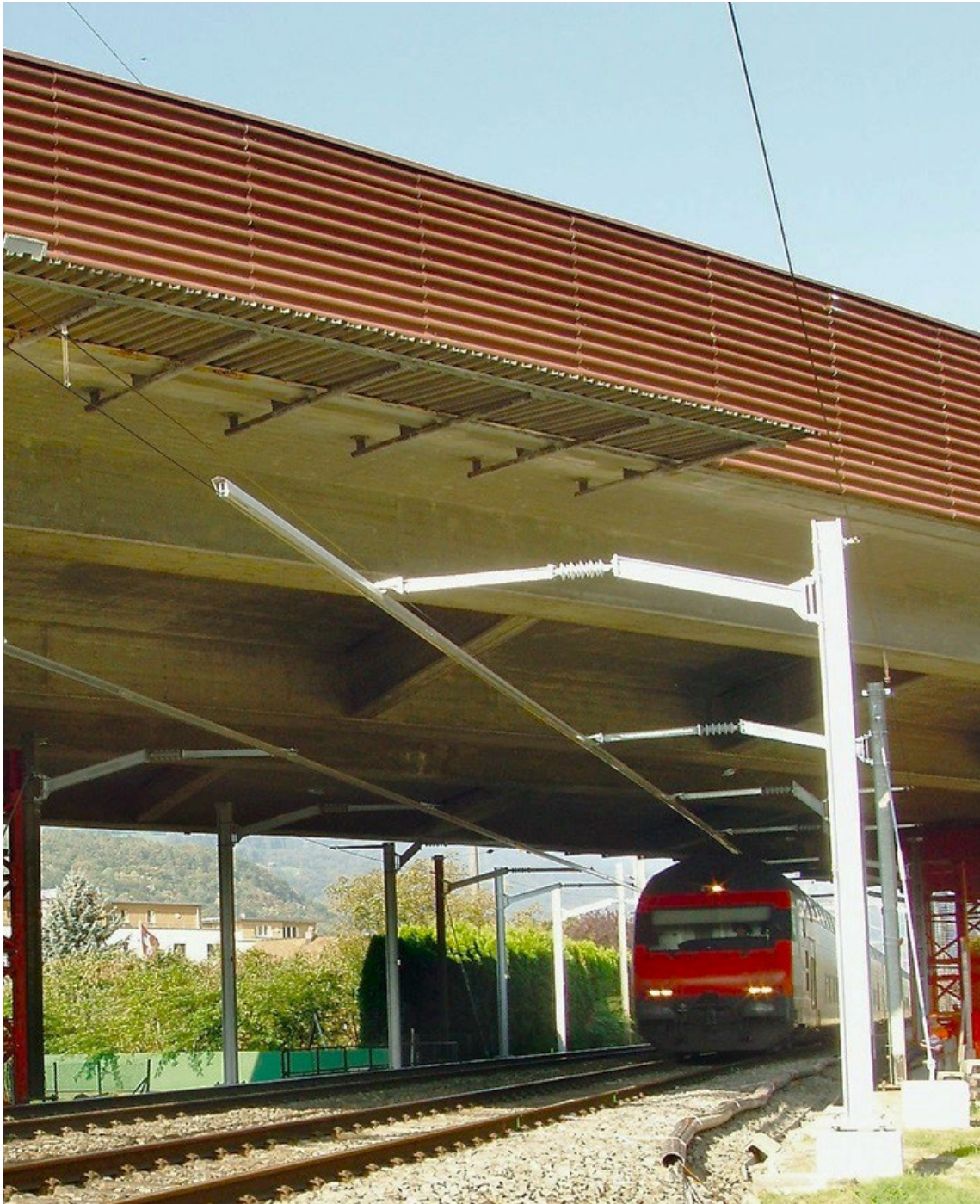
Conductor bar on a European OCS system passing under a low bridge (photo: Furrer+Frey)
