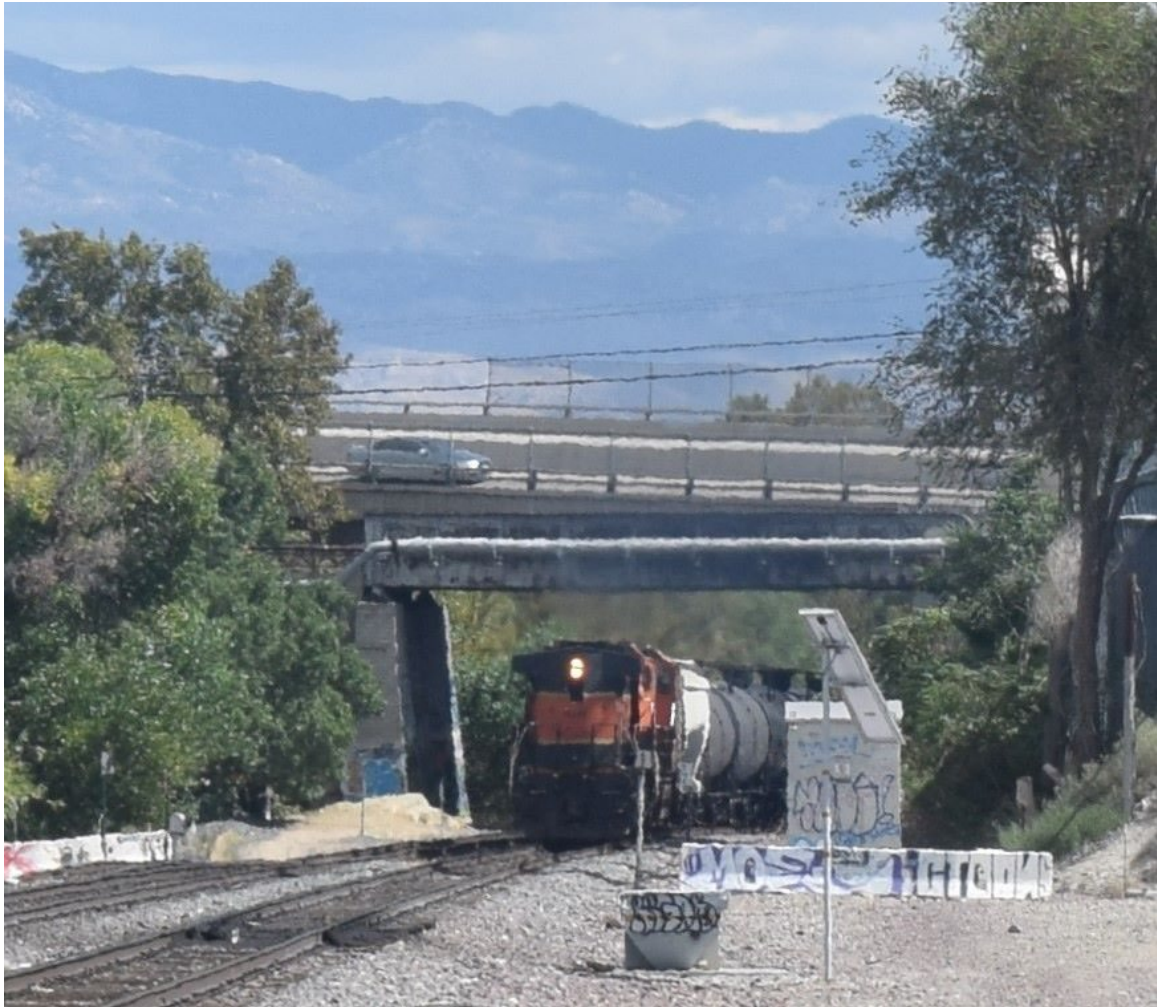
Mineral Road [23.6'] and D Street [24.9'] bridges, Victorville (September 15, 2023 photo)
